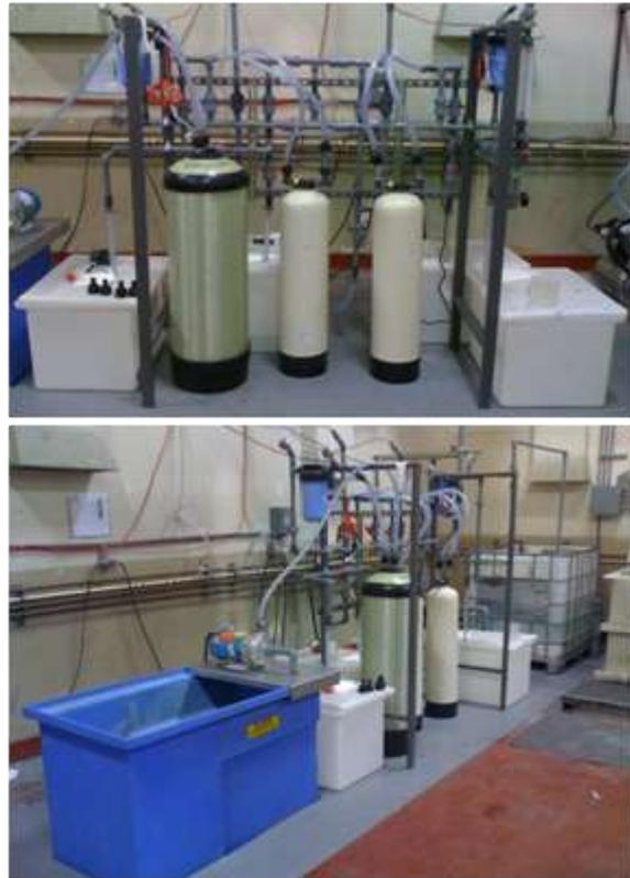
The new ion exchange system is safer, eliminated the "Swamp" and the raised storage tank, and reduced the use of floor space.
